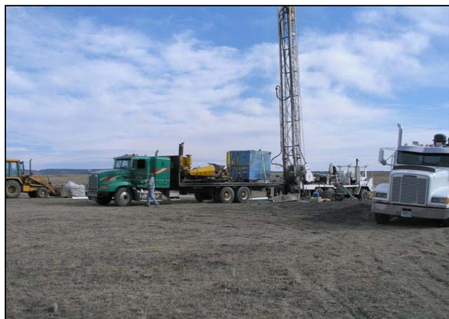
Photo 2.4 – Powertech 2007 exploration drilling.
