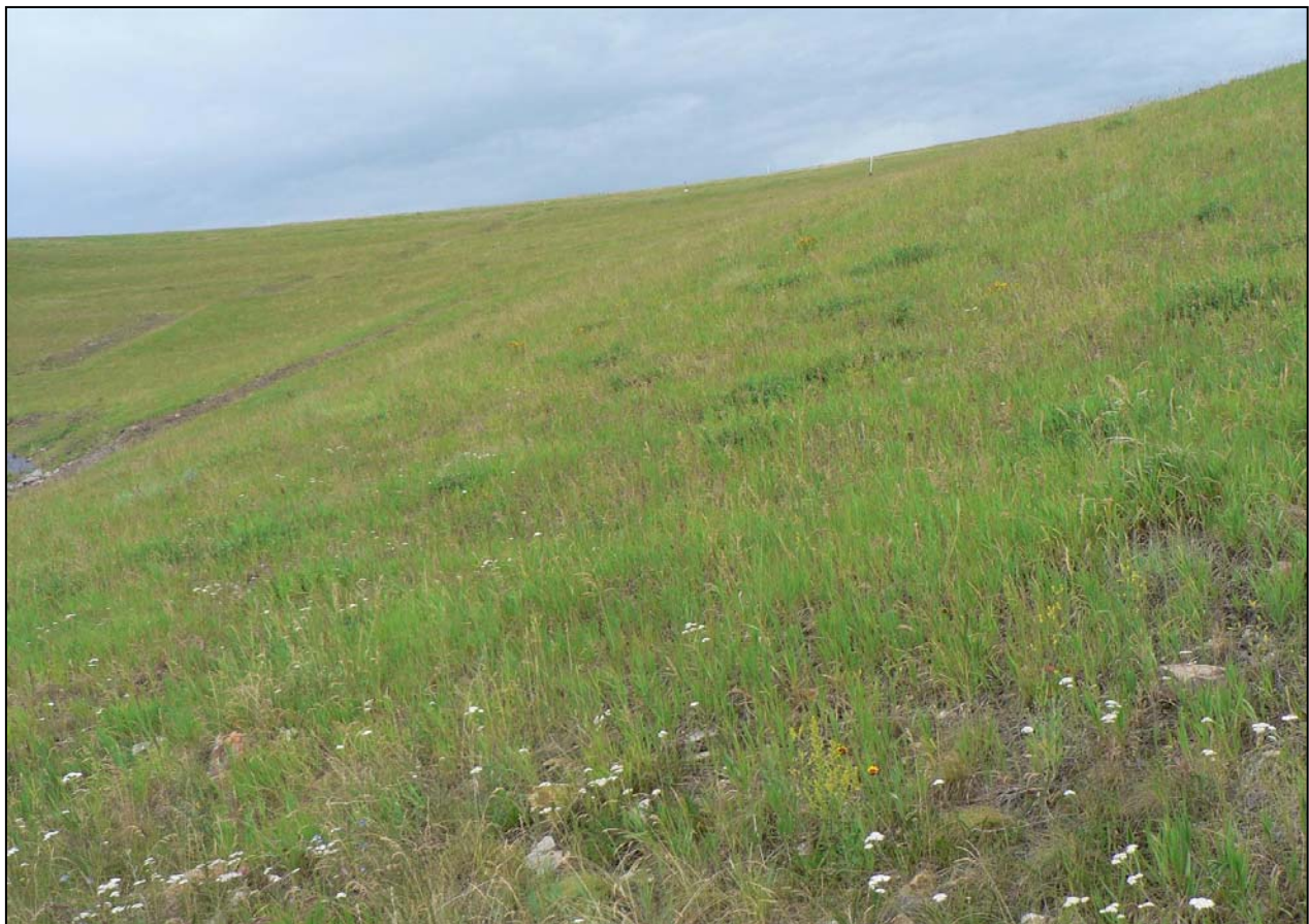
Photo 1.5 – Reclaimed pit impoundment slope at the Richmond Hill Mine.
