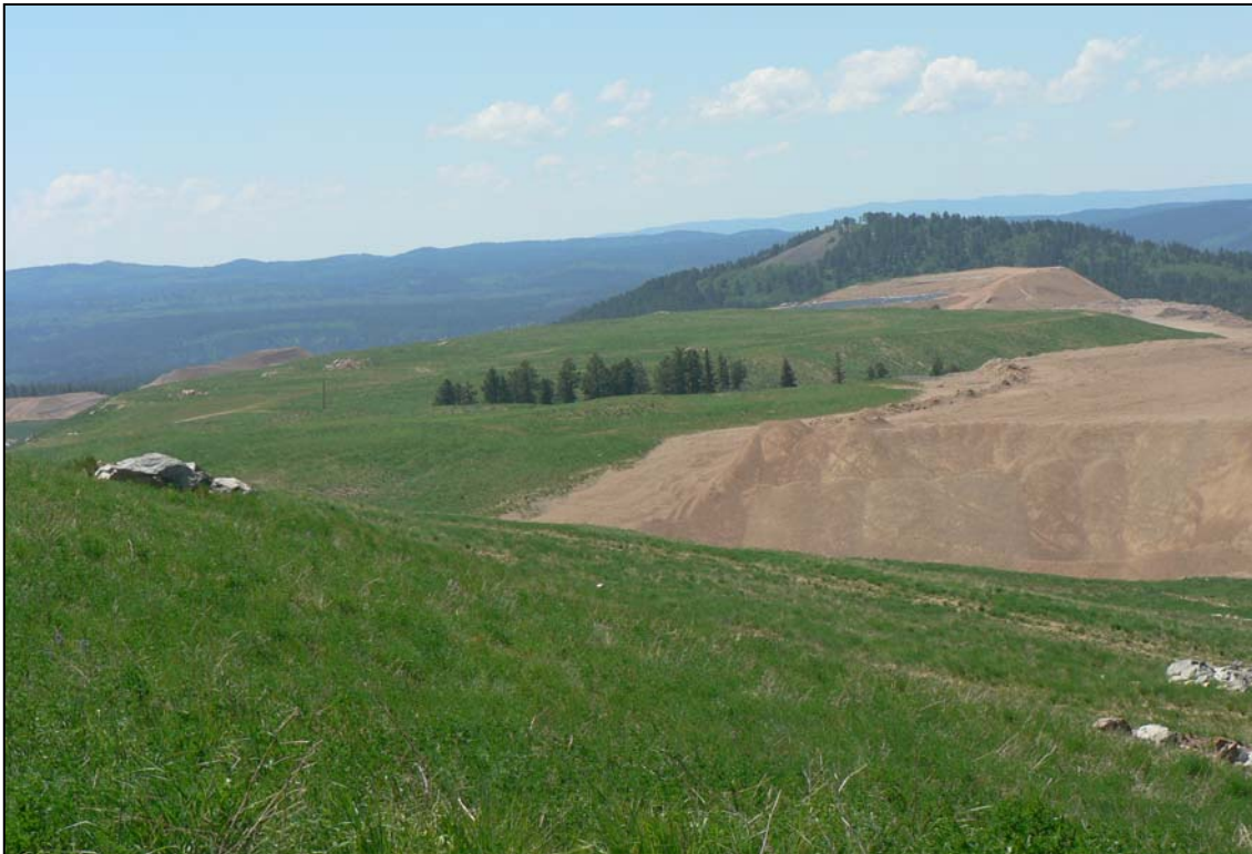
Photo 1.6 – Concurrent reclamation completed on backfilled Portland Pit (foreground) and on Reliance Depository (background) at the Wharf Mine.
