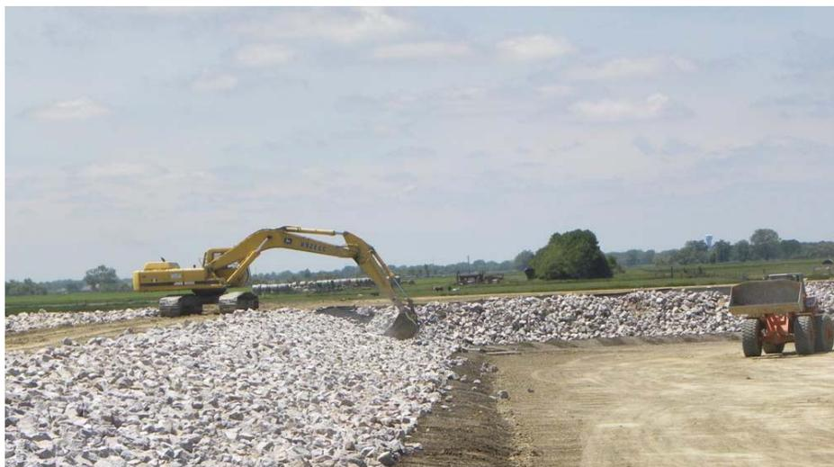
Placing rip rap on the berm of a new cell at the Aurora wastewater treatment facility.
