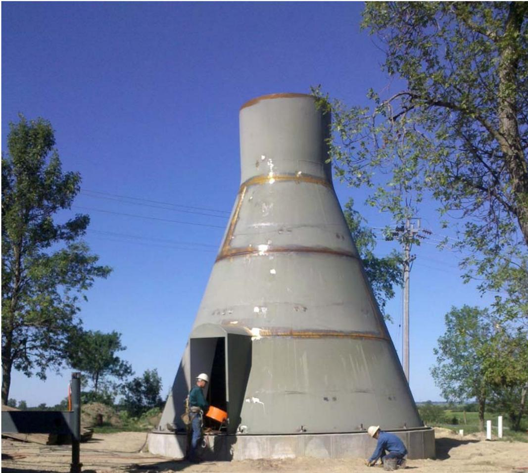
Construction of a 200,000-gallon water tower for the Hanson Rural Water System.
