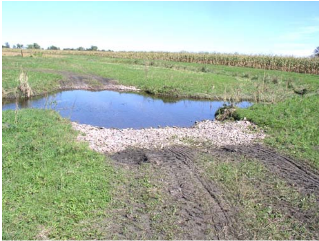
Figure 6a. Rock Crossing.
