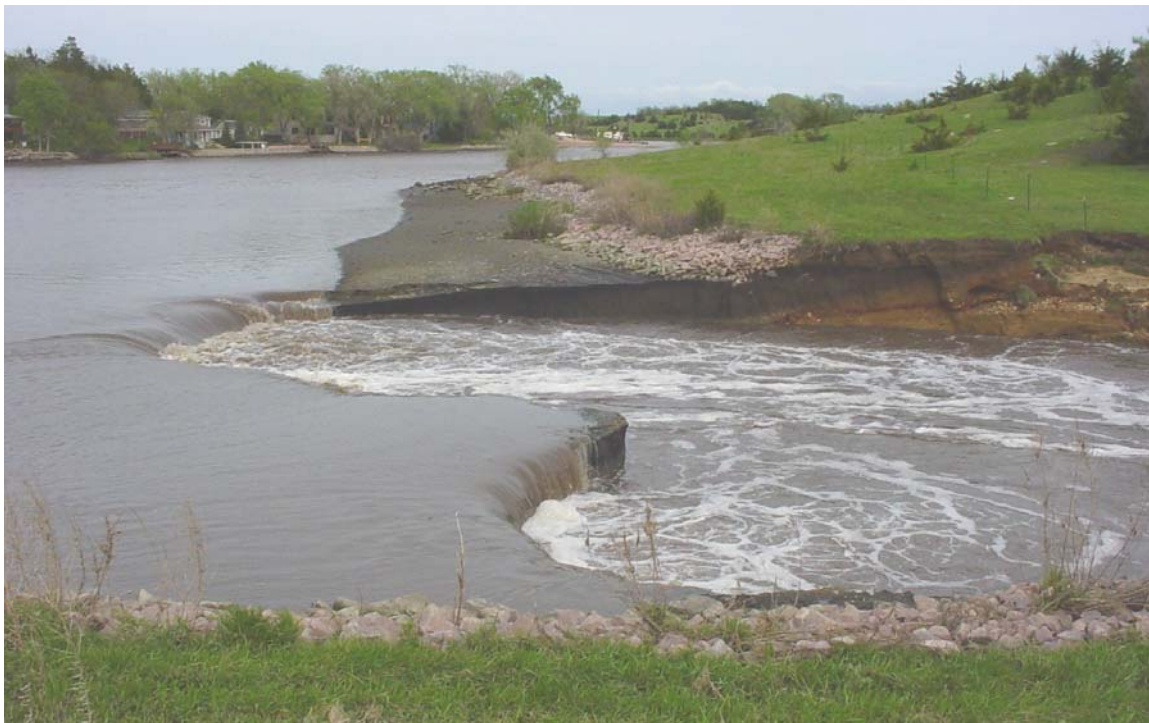
Figure 5: The emergency spill way after breach, spring 2007.
