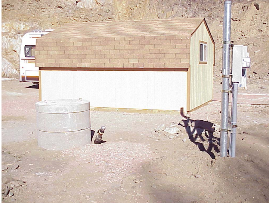
Figure 8. Wellhead of Keystone Well #4. Plumbing into the shed has been completed.
