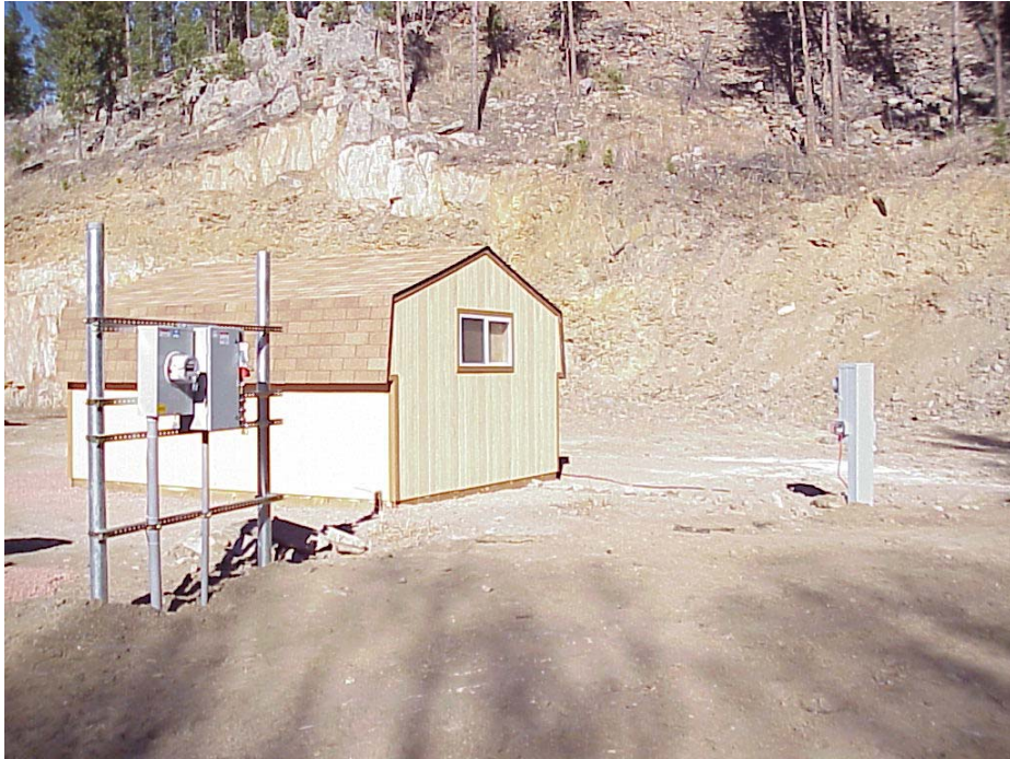
Figure 7. Shed and power installation at Keystone Well #4.
