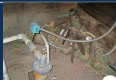
Seal on wellhead not watertight
