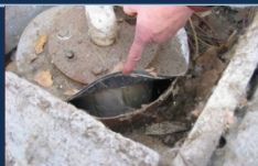
Seal on wellhead not watertight
