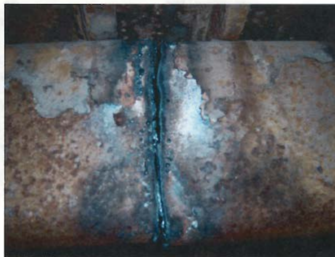
Photo #4: Chassis rail cut in half
