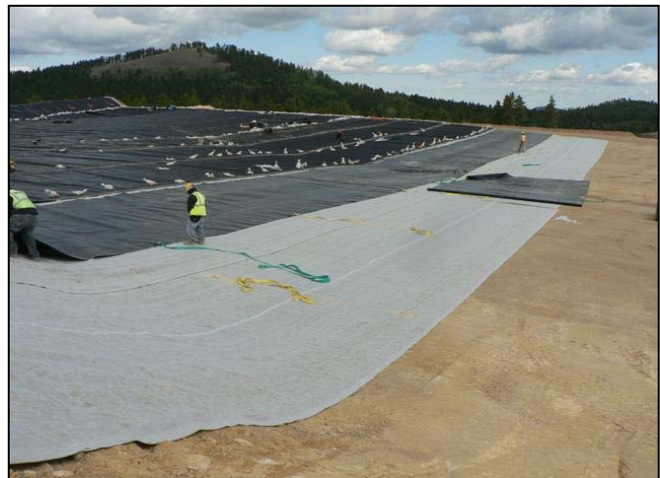
Photo 1.2 – Wharf Pad 5 construction.
