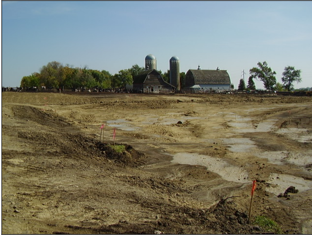
Figure 3: VTA system under construction 9/25/2008.
