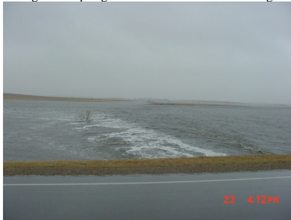
Figure 3: Spring Creek Main Channel Flooding
