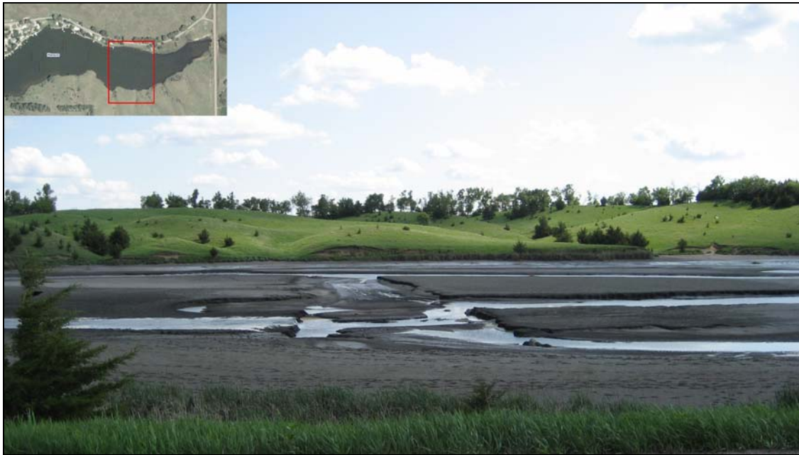
Figure 6: Area of dredging after spillway breach, and lake drained.
