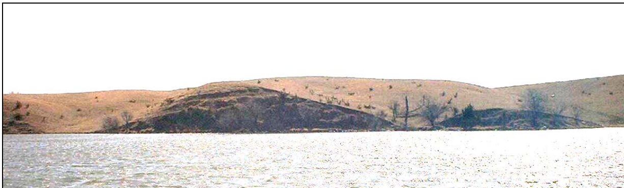
Figure 8: Area along the south shore of Lake Hanson before stabilization.
