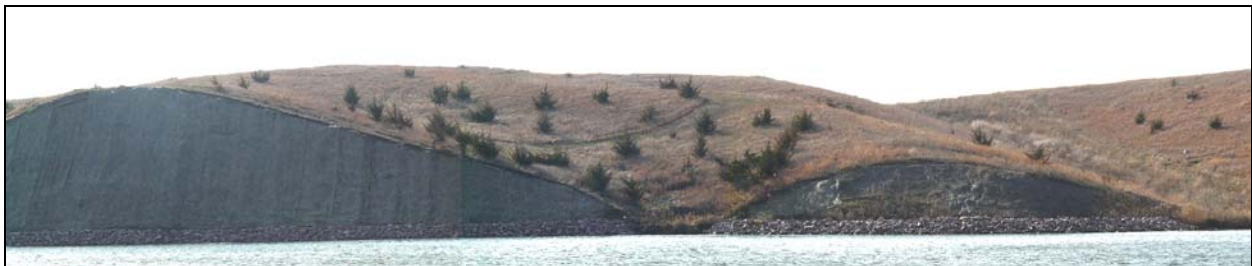
Figure 9: Area along the south shore of Lake Hanson after Stabilization.
