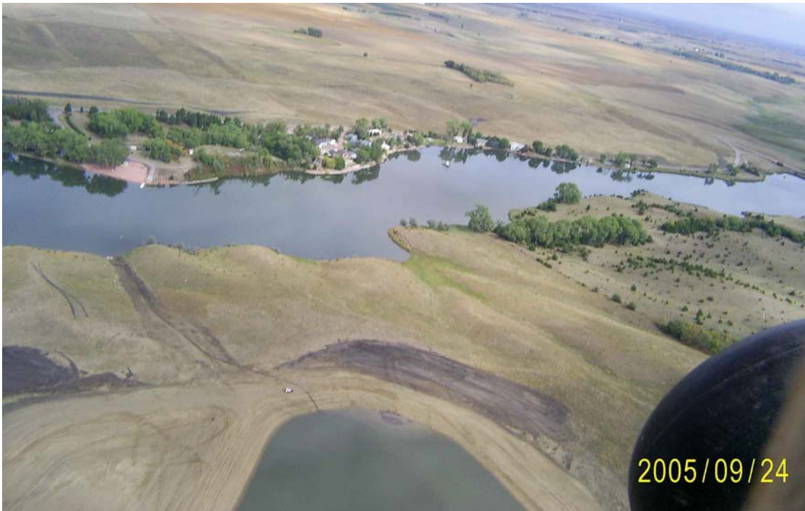
Figure 4: Start of the dredging project.
