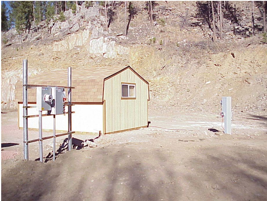
Figure 7. Shed and power installation at Keystone Well #4.
