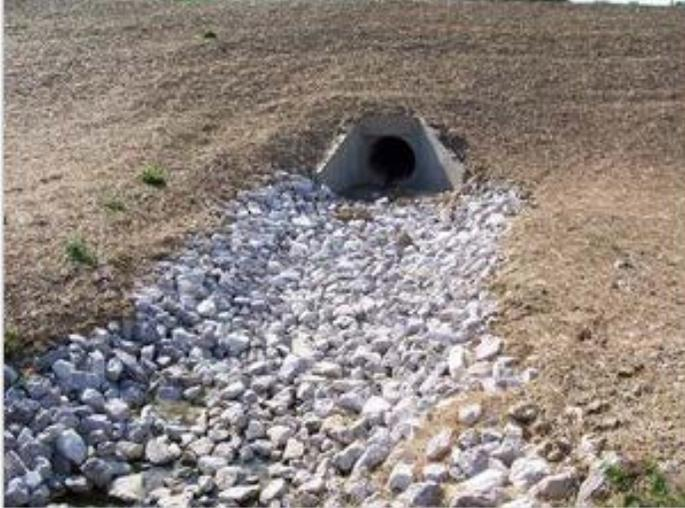
[https://stormwater.pca.state.mn.us/index.php?title=Sediment\\_control\\_practices - Outlet energy dissipation](https://stormwater.pca.state.mn.us/index.php?title=Sediment_control_practices_-_Outlet_energy_dissipation)
